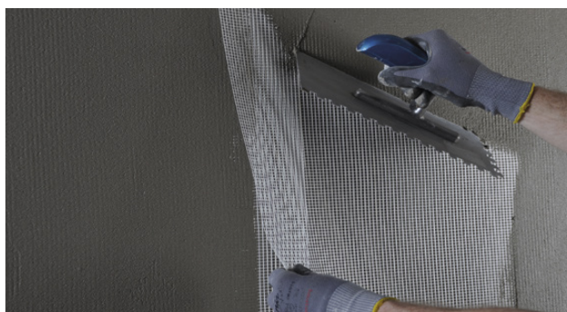
Montering af net med min. 10 cm overlap
