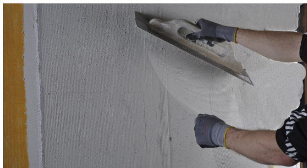
Montering af net med min. 10 cm overlap
